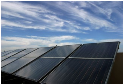
Figure 1: PV plant (source: microsoft)
